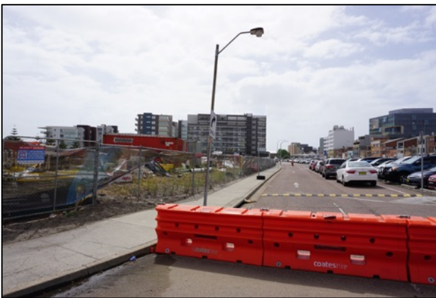
FIGURE 27: VIEW EAST ALONG WRIGHT LANE, BETWEEN SITE 1, AND SITES 2 AND 3 (SOURCE: CURIO 2018)
