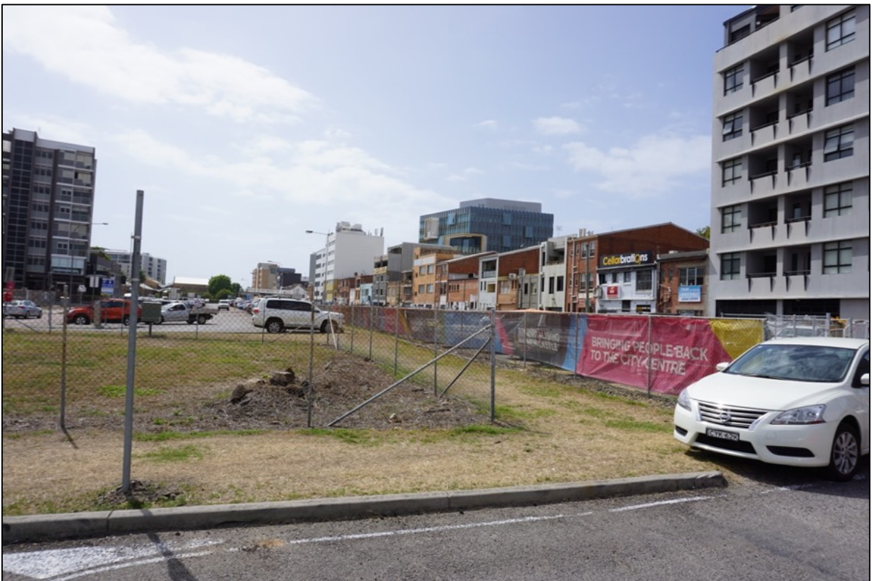
FIGURE 19: VIEW EAST FROM WORTH PLACE ACROSS SITE 2, CARPARK TO LEFT, FORMER RAIL LINE TO RIGHT (SOURCE: CURIO 2018)
